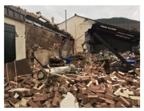
A Health and Safety Executive (HSE) investigation found Rathburn Chemicals had an inadequate system in place which failed to control the amount of steam and heat being generated during its distillation process. The company also failed to adequately detect any signs of overheating which could lead to flammable vapour being ignited.
