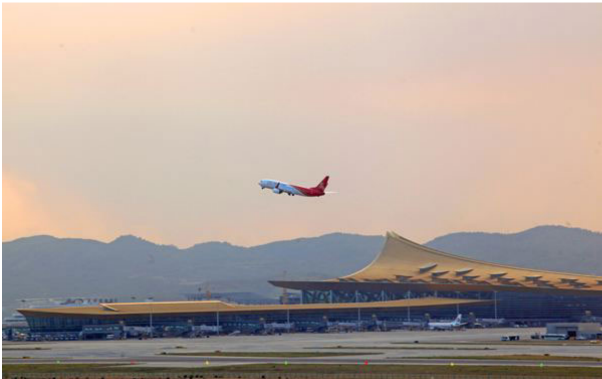
Changshui International Airport in Kunming, Yunnan Province. [Photo: China Daily]
