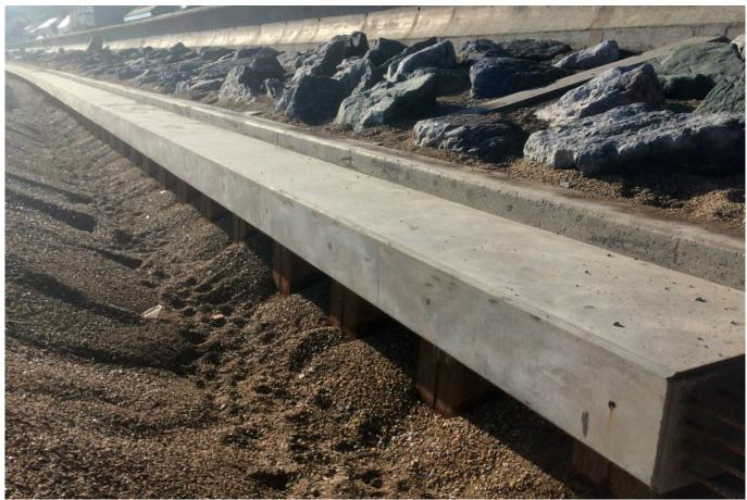
Steel sheet piles have been driven in front of existing piles and topped with concrete beams
