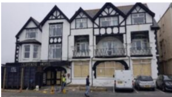
The former Cliffdene Hotel in Newquay
