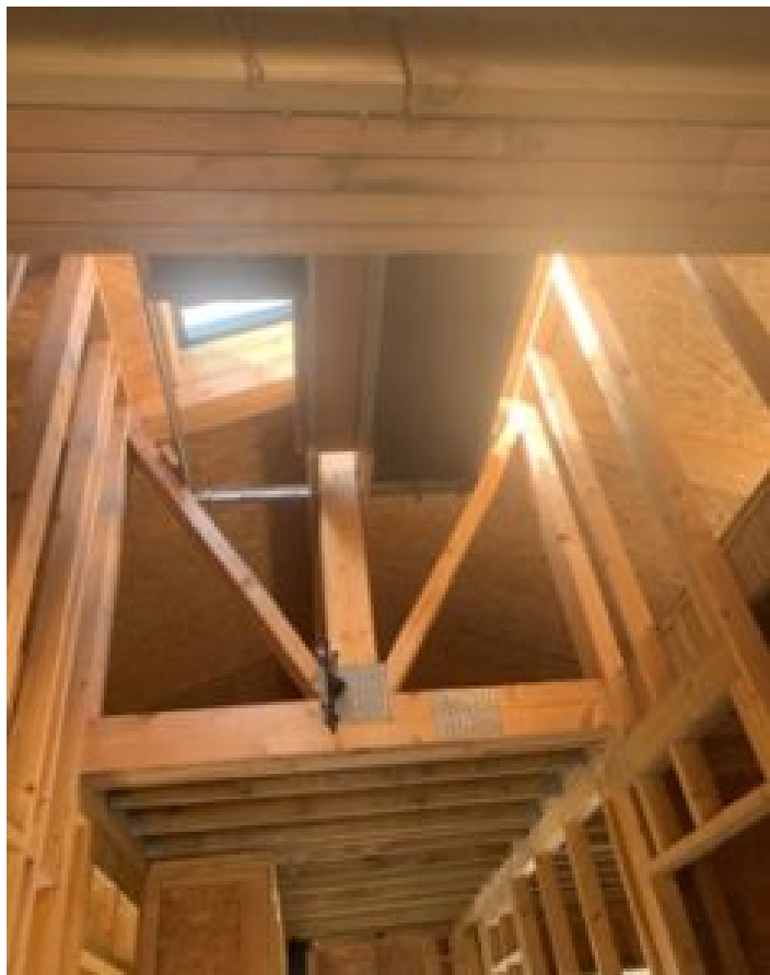
View of the roof inside the property
