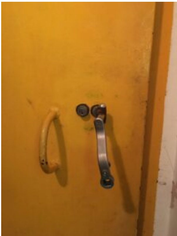
The door to the company's industrial radiography enclosure
