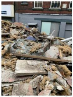
• Significant amounts of asbestos-containing debris to the front and rear of the building and along the public highwayconstructio
