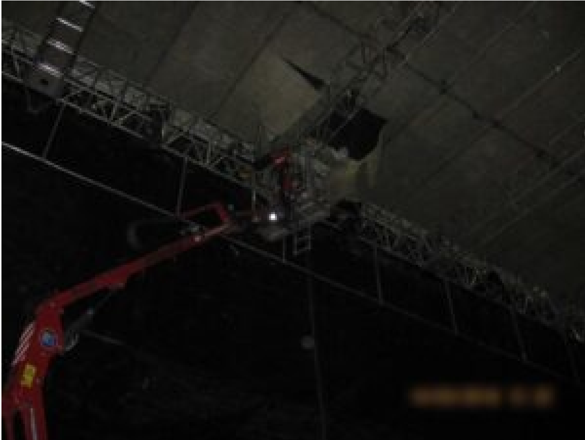
The roof which Mr Bowry was working on
