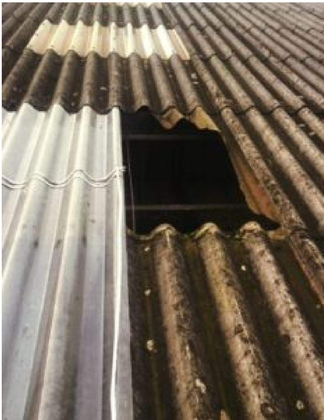
The roof Billy had been working on
