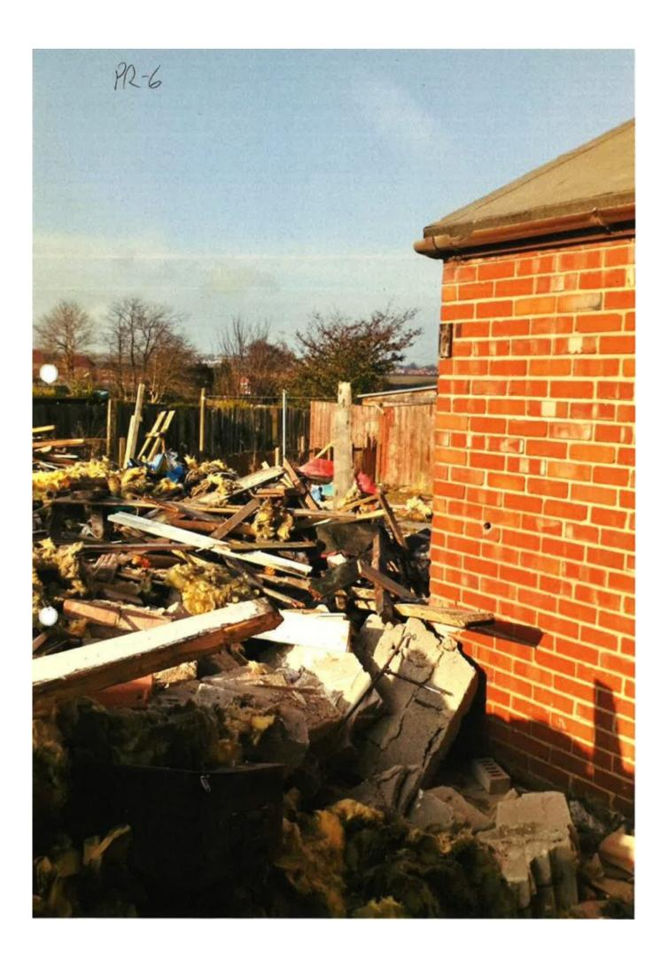
An investigation by the Health and Safety Executive (HSE) found that the company failed to suitably ensure that demolition work within its grounds was carried out in such a manner as to prevent danger. The work had not been thoroughly planned to ensure that demolition waste was fully enclosed within the site boundary, and there was no secure fence to prevent unauthorised access to the site.
