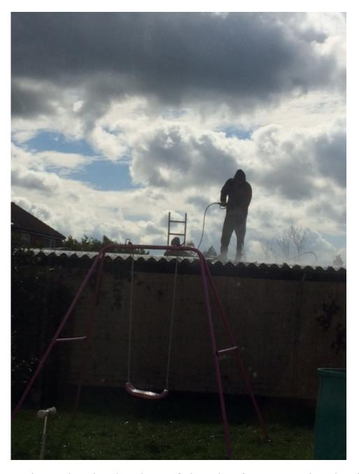
An investigation by the Health and Safety Executive (HSE) found that work should have been planned to include the use of basic precautions as detailed in published and widely recognised guidance for working with asbestos cement. Low energy cleaning methods and proper protective measures would have prevented the release of asbestos fibres thus eliminating much of the risk.
