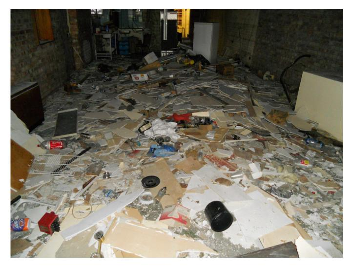
An investigation by the Health and Safety Executive (HSE) found that a management asbestos survey and a refurbishment and demolition asbestos survey had not been completed prior to the work starting, and the work had not been completed by a licenced asbestos contractor.
