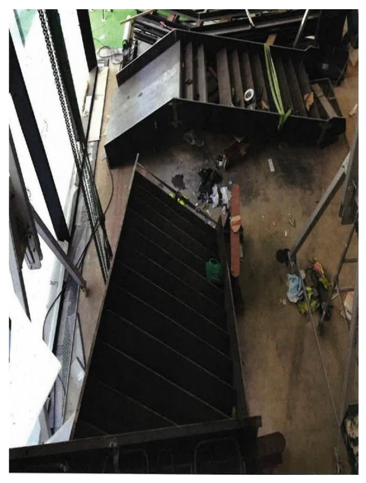
An investigation by the Health and Safety Executive (HSE) found that Leyton Group Construction Ltd failed to properly plan the lifting operation. The lift plan was not specific to the job and the method statement lacked the level of detail required about the load, how it should be slung and how it
