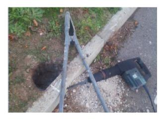
While operating the electric breaker, one of the operatives struck an 11kv electricity cable causing a large flash and engulfing him in flames. The operative sustained serious burns to his face, chest, abdomen, groin, both arms and both legs, amounting to approximately 50% total body surface area burns.
