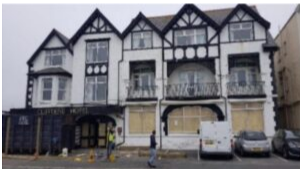
The former Cliffdene Hotel in Newquay
