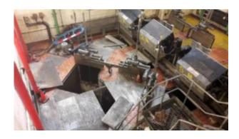
Edinburgh Sheriff Court heard how, on 9 June 2017, an employee of Scottish Water entered into the screen well area at Prestonpans Pumping Station and fell through the insecure floor panels into a sewage filled storm channel some 3.1 metres below.
