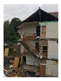
A building contractor was prosecuted after carrying out unsafe excavation works, which resulted in the partial collapse of a residential building.
