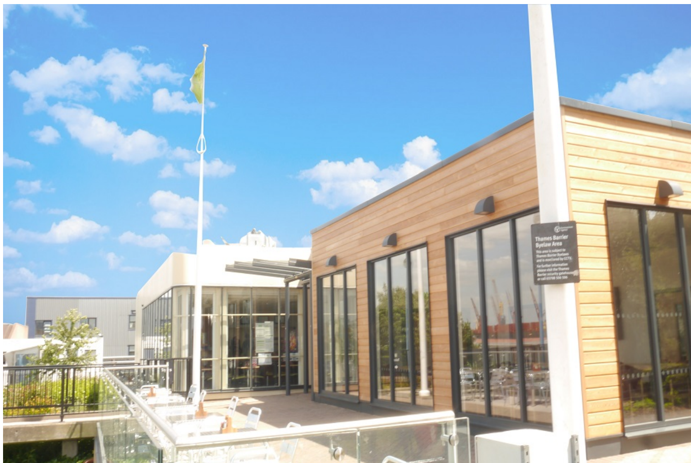
New Thames Barrier cafe and information centre
