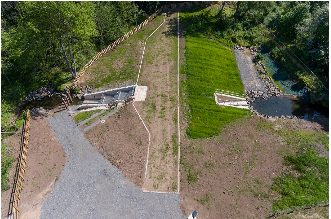
Cotting Burn dam aerial image
