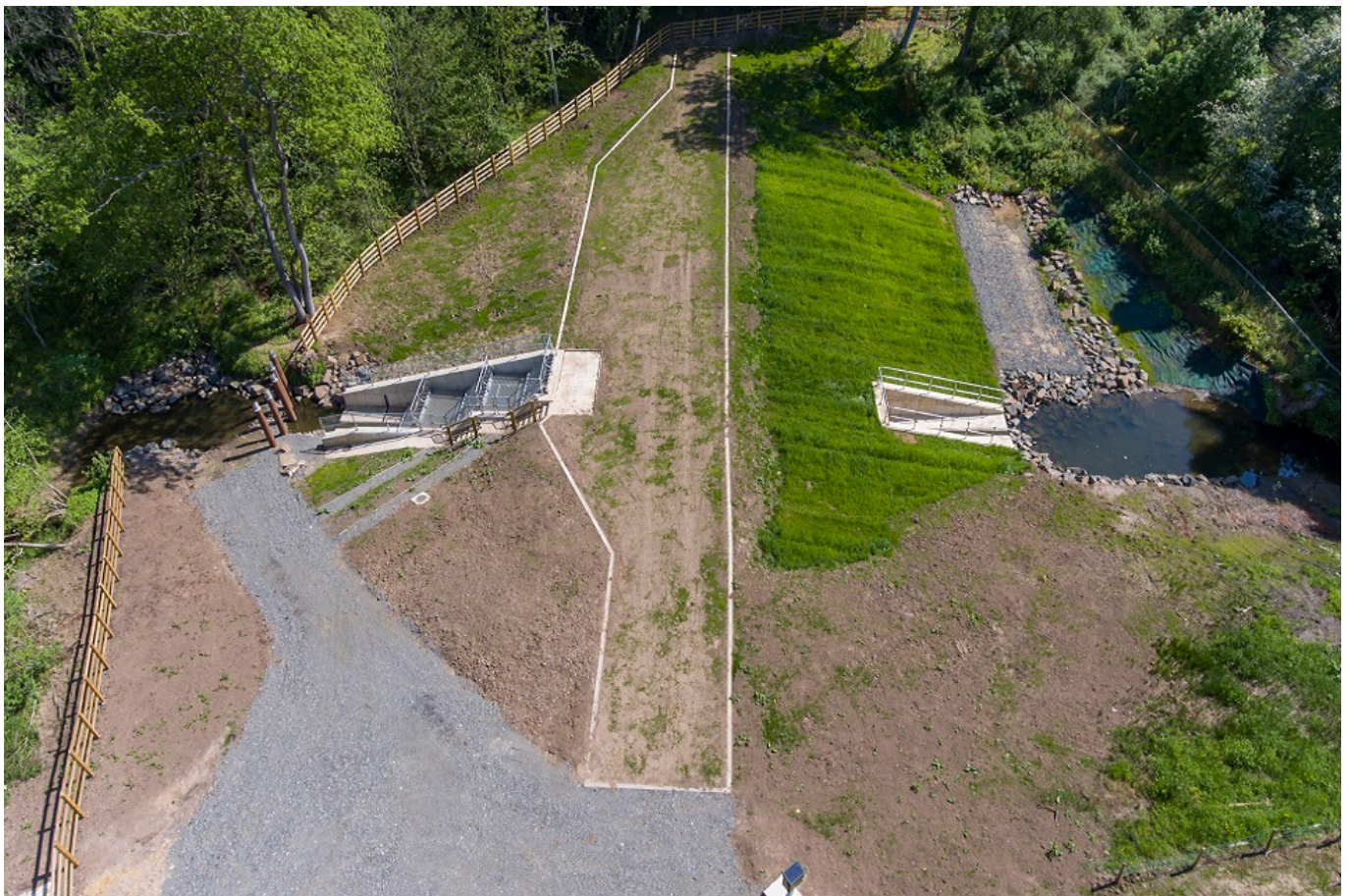
Cotting Burn dam aerial image
