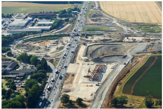
The abutments for the two new bridges can be seen just south of the existing bridge and further down on the right of the road, the bridge decks are under construction
