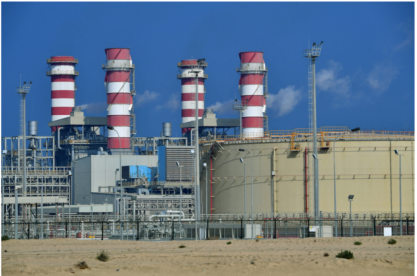
A view of Jubail Desalination Plant at the Jubail Industrial City, about 95 kilometers north of Dammam in Saudi Arabia's eastern province. (AFP/File Photo)
