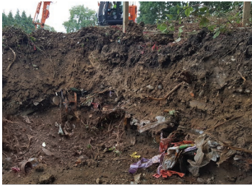
BEFORE - examples of the excavated material and accumulated rubbish found on sites being developed by welters, unsuitable for earthen burial
