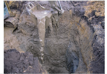
BEFORE - examples of the excavated material and accumulated rubbish found on sites being developed by welters, unsuitable for earthen burial
