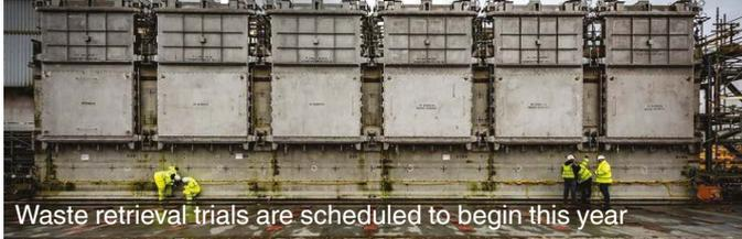
Engineering teams have installed equipment to scoop up and remove material from Sellafield's Pile Fuel Cladding Silo.
