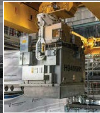
The 50-tonne package was safely placed onto a machine that will grab waste out of the building
