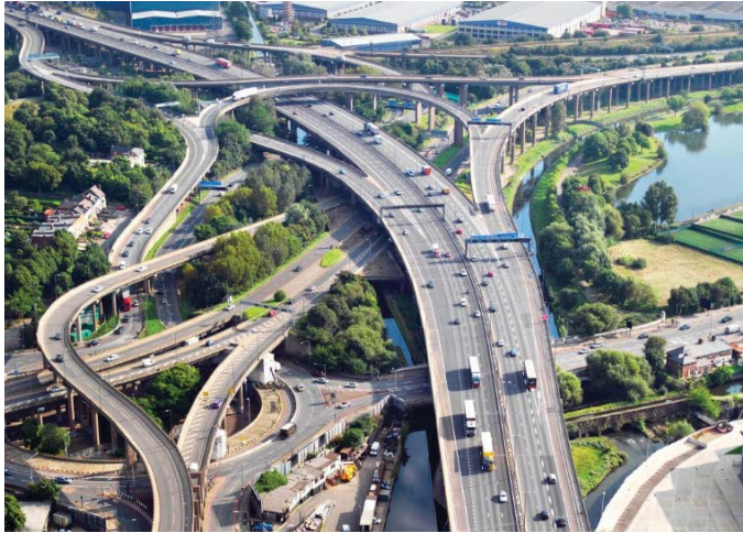
Aerial view of Gravelly Hill Interchange, w: Birmingham a.k.a. Spaghetti Junction, by Highways Agency photo
